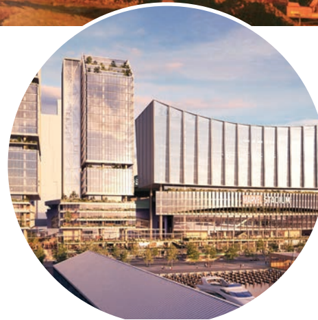
▲ A render of the AFL's plans for the redevelopment of Marvel Stadium's waterfront edge.
